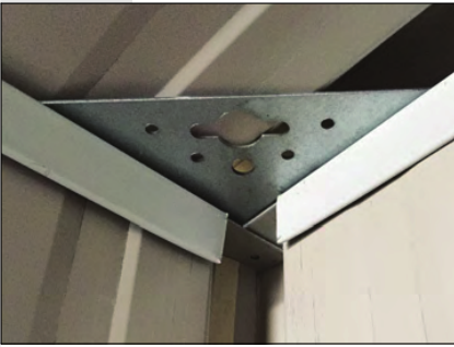
Corner Anchor Interior - Top
