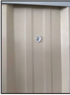
rivets with washer
